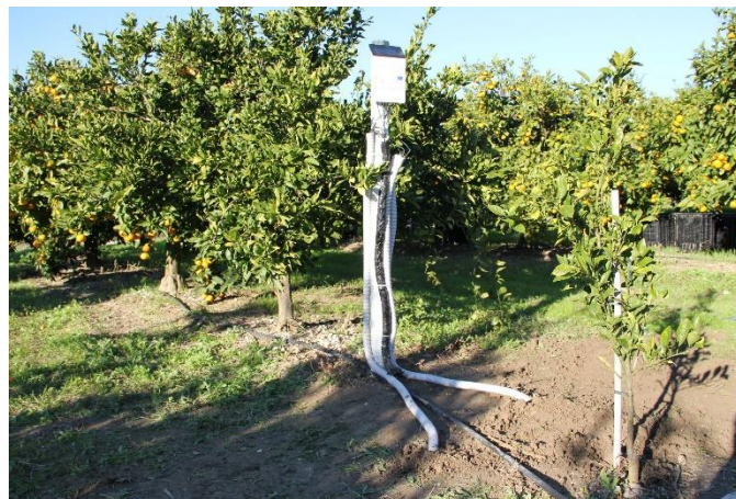
Installed soil monitoring system
