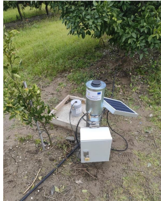
MPP — ground water
